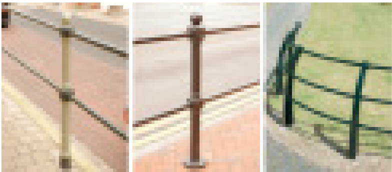
Cast iron balustrades
