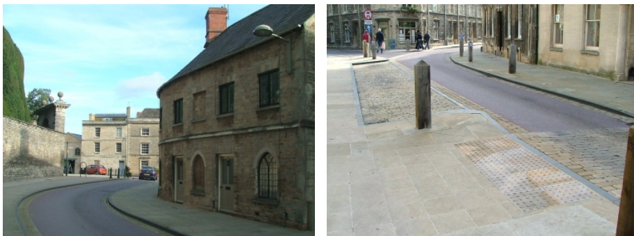
Photos 7.1 and 7.2: Redesigned highway resolves traffic issues while improving the townscape
