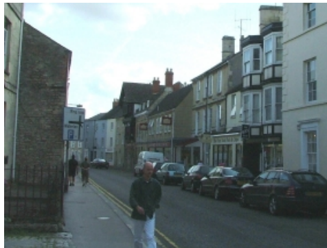
Photo 8.24: Predominantly older buildings at eastern end of Dyer Street
