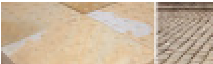
Natural stone tactile paving; reclaimed Yorkshire setts
