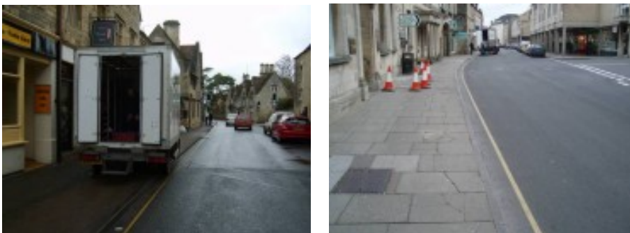
Photos 3.15 and 3.16: Obstruction and damage to footpaths - Cricklade Street and Dyer Street
