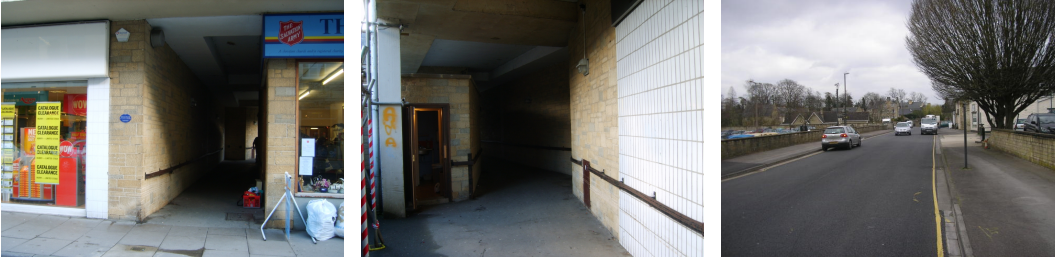
Photos 7.15 - 7.17: Poor pedestrian linkages between Dyer Street and The Waterloo car park
