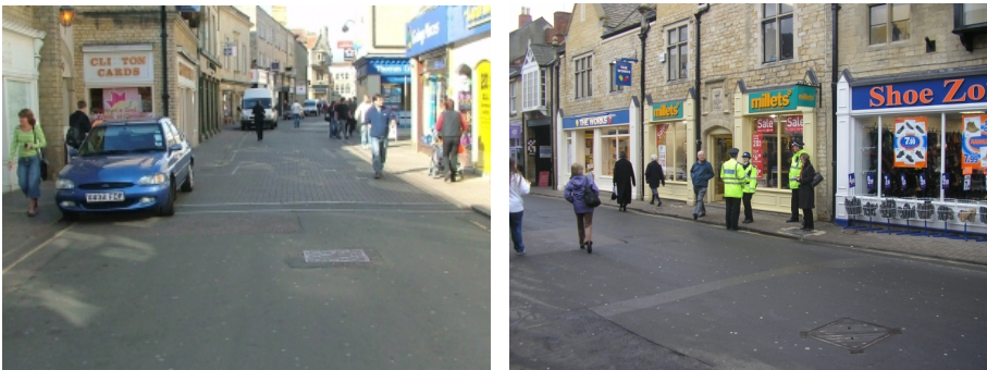
Photos 8.12 and 8.13: Poor quality paving and streetscape in Cricklade Street
