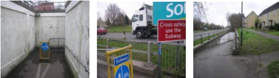
Photos 5.22 - 5.24: Pedestrian subways under the 'ring' road
